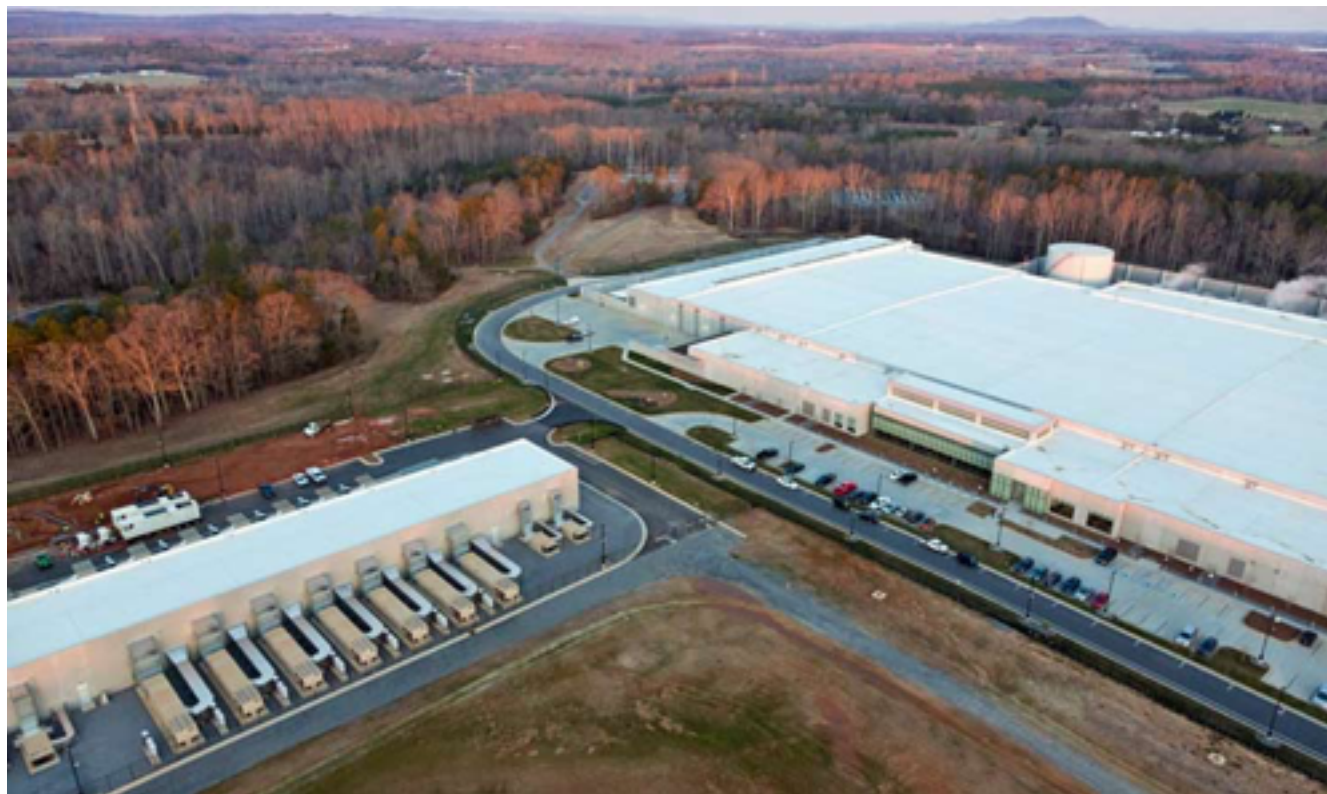
The home of the iCloud: The Apple data center campus in Maiden, North Carolina, featuring a massive 500,000 square foot building (at right) supported by a smaller “strategic” data center using modular data center technology. (Photo: Apple)
